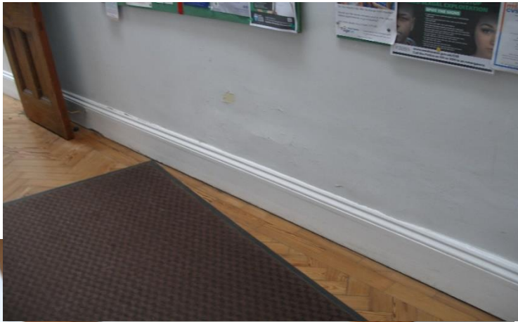
Front section, North facing wall.
