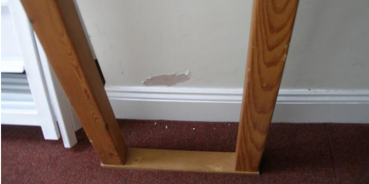
Rear section, North facing wall, opposite the doors to the hall.
